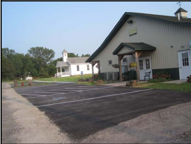
Macadam for parking and new sidewalk
